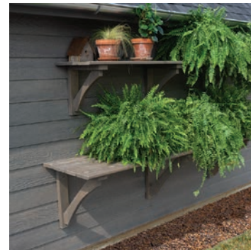
Exterior Plant Shelves Set of two, 16" and 22", 5/4" treated shelves with arched timber braces below.
