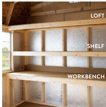
Loft, shelf, workbench Lofts and shelves are 7/16" OSB. Lofts come in 24"D sections, installed at top of wall. Shelves are 16"D, installed at 18", 34" or 54". Workbenches are 24"D 3/4" SmartFloor with backsplash and rounded front, installed 35" high, below windows.
